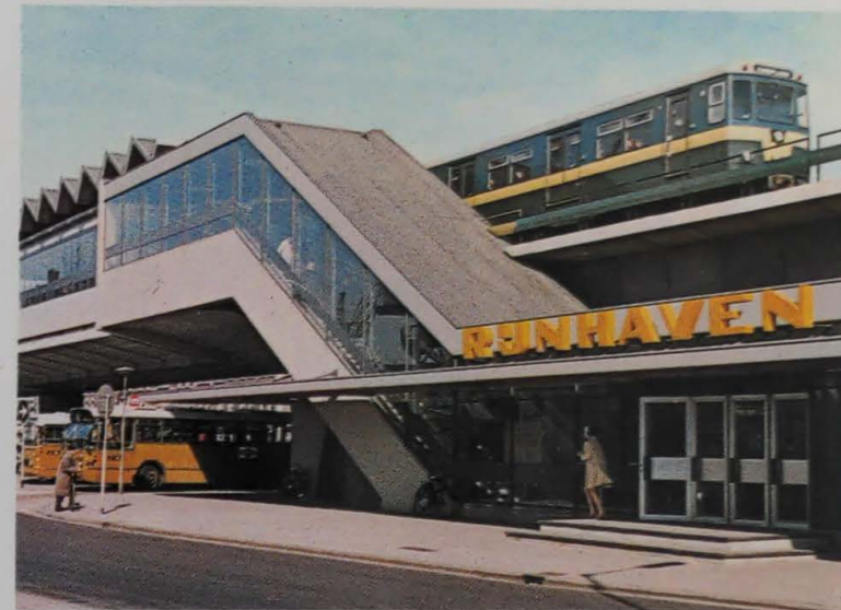
Feeder bus services to rail terminals are a vital part of the balanced transport system envisaged for Melbourne. Here is a typical modal exchange station of the future.
