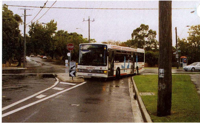
Left turning bus impeded by raised island and signs
