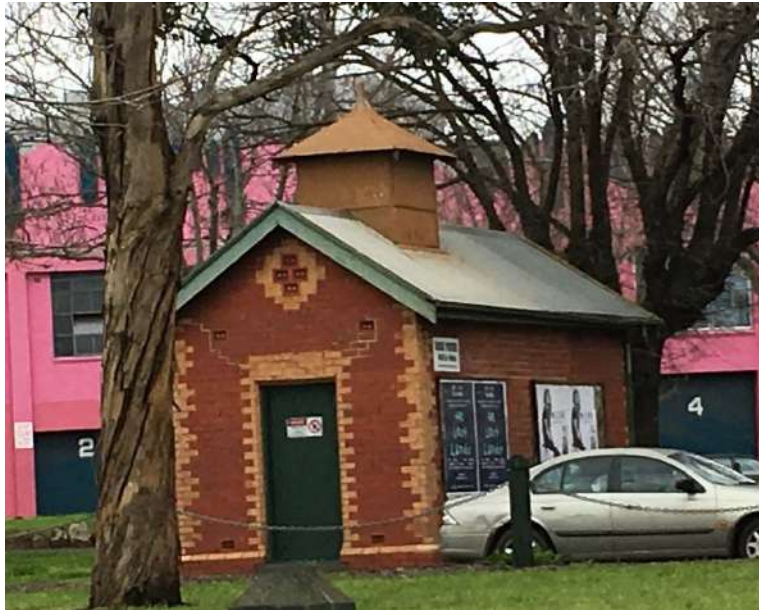
Figure 110. Electrical substation at the corner of Alexandra and Queens parade, Fitzroy North. (Context, 2016)
