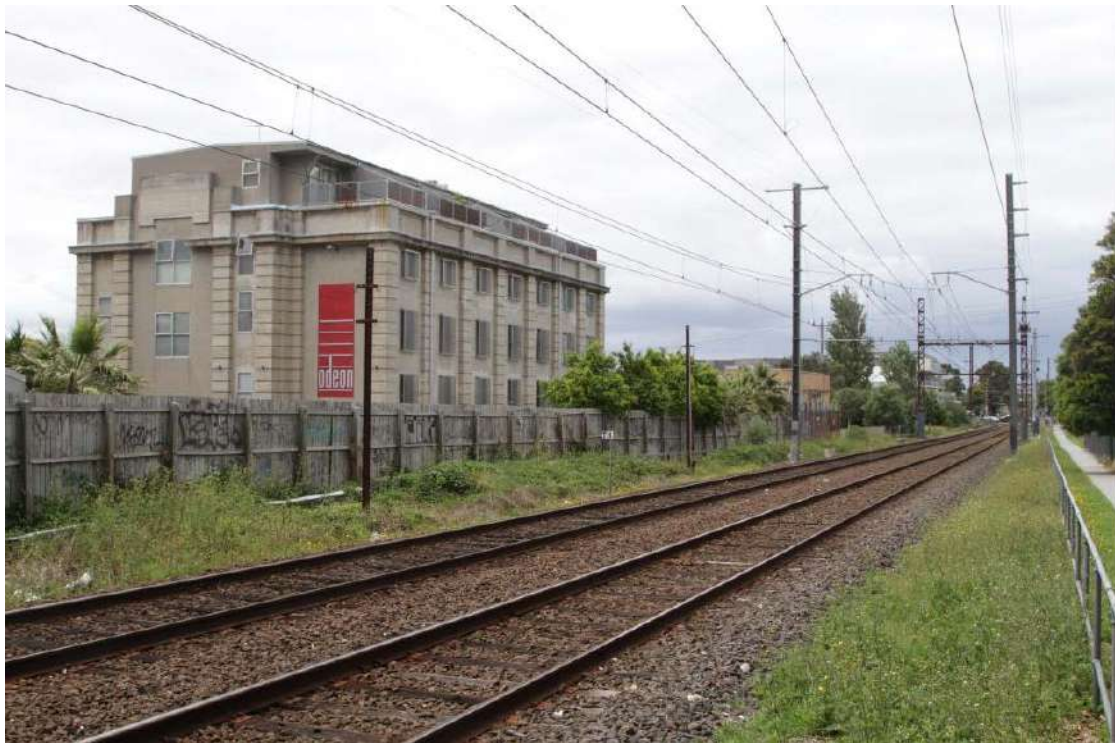
Figure 153. Mentone Substation, 2-10 Teague Avenue, Mentone, 1921-22, by J.W. Harding (architect). (Source: Wong 2016).
