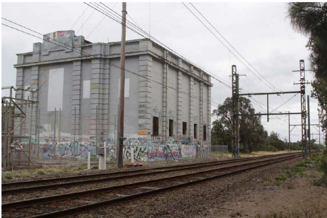
Figure 154. Seaford Substation, 28F Station Street, Seaford, 1925, by J.W. Harding (architect). (Source: Wong 2016).
