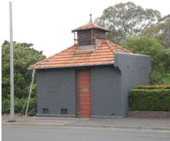
Substation at 190A Canterbury Road, Canterbury.
