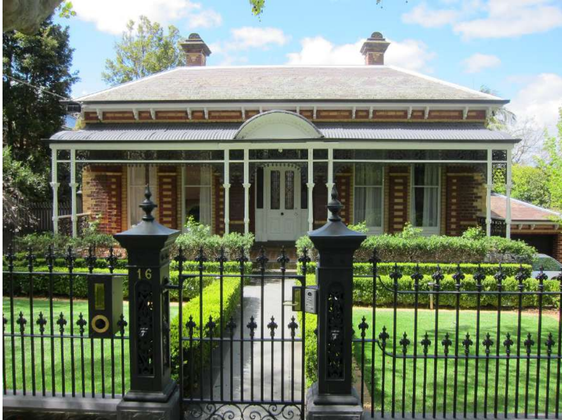
Figure 54. Number 16 Victoria Avenue. (Source: Context, 2016)
