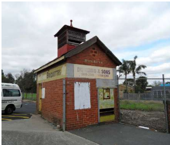
Substation at 6 Harp Road, Kew.
