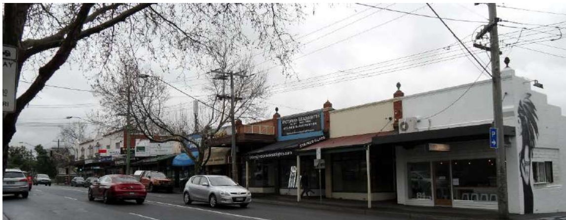
Figure 4. Western end of the precinct and the row of 1909 shops.
