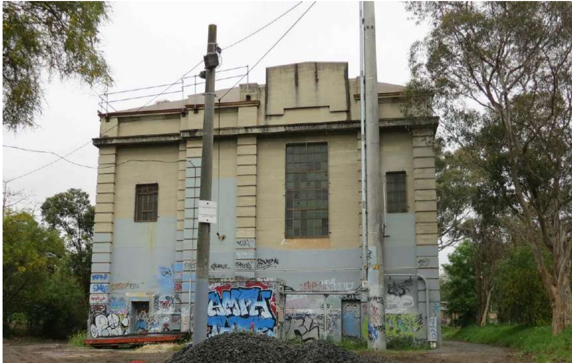
Figure 150. View of the east elevation of the East Camberwell substation, looking north-west. Apart from variations in fenestration, the elevation is a mirrored facsimile of the west elevation of the building. (Source: Trethowan Architecture, 2016)
