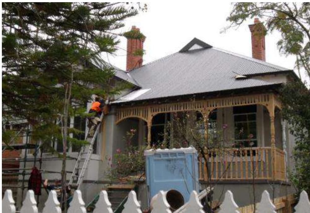
Figure 17. 6 Dudley Parade undergoing works in September 2016 (Source: Context, 2016)
