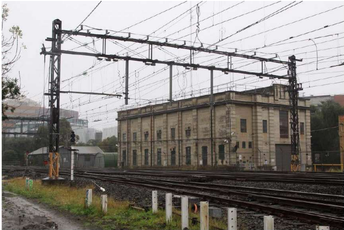
Figure 152. Caulfield Substation, 98 Queens Avenue, Caulfield East, 1921, by J.W. Harding (architect). (Source: Wong 2016).
