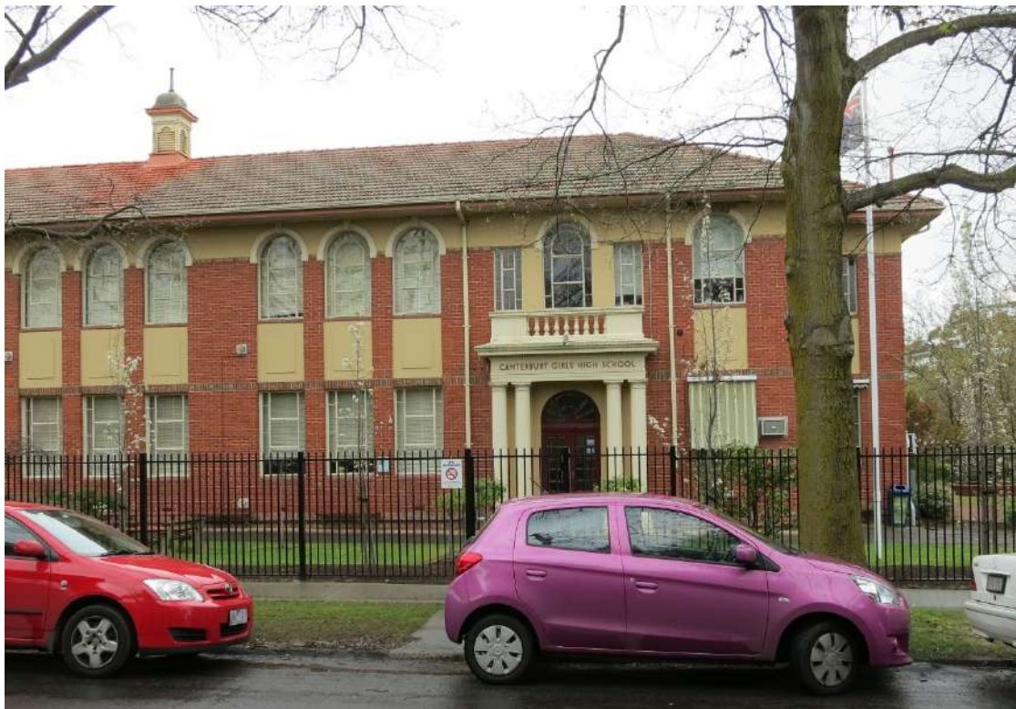
Figure 125. View of the main entrance to Canterbury Girls' Secondary College from Irlbarra Road, looking south. Note the extant semi-glazed dual doors with overhead fanlights to the entrances and Palladian style tri-partite window arrangements above the porticos. (Source: Trethowan Architecture, 2016)
