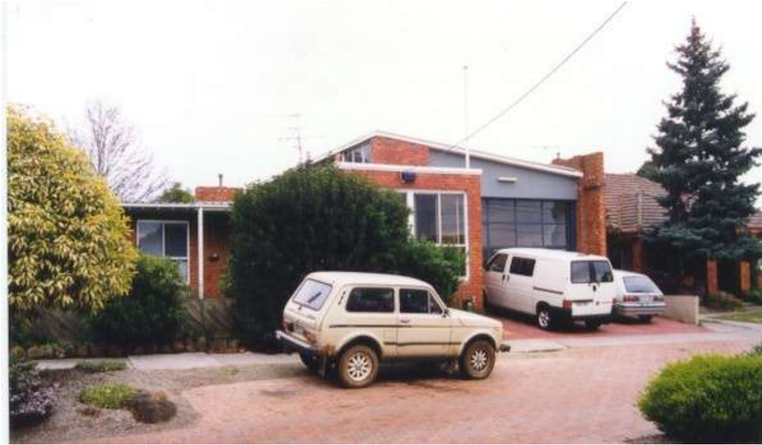
Figure 81. Former Ringwood Ambulance Station of 1955 (Source: City of Maroondah, 1999)
