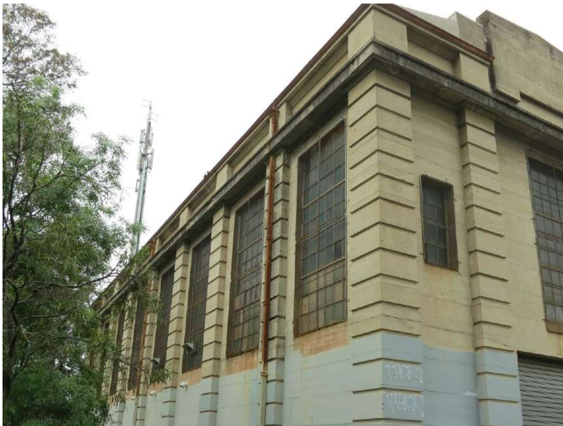
Figure 151. View of the north elevation of the East Camberwell substation, looking south-east. The height and extent of glazing are indicative of a double-height space on the interior of this part of the building. (Source: Trethowan Architecture, 2016)
