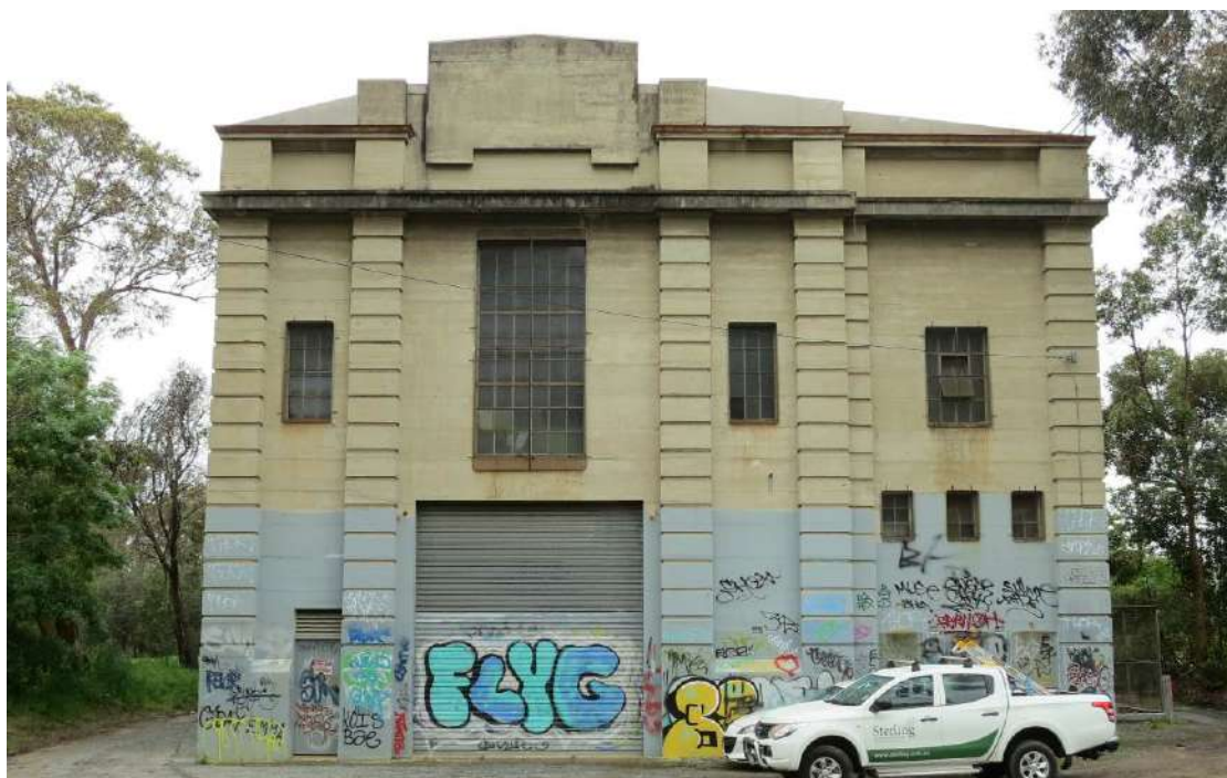
Figure 149. View of the west elevation of the East Camberwell substation from Boroondara Park, looking south-east.
