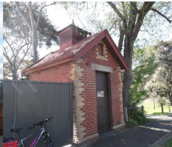
Substation at 26A Myrtle Road (next to 37 Canterbury Road), Canterbury.
