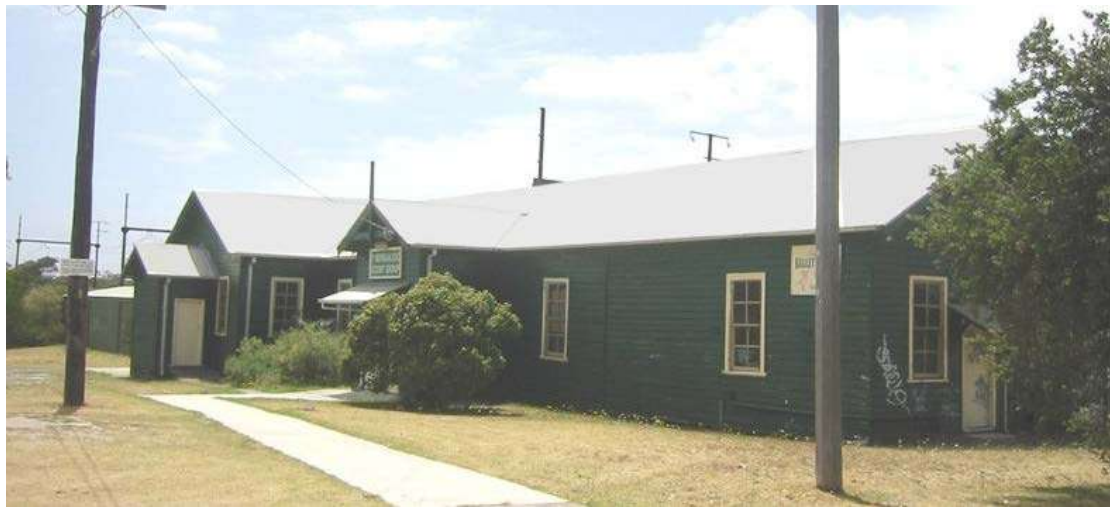
Figure 166. 1st Mordialloc Scout Hall, 429 Nepean Highway, of 1914. (Source: City of Kingston)
