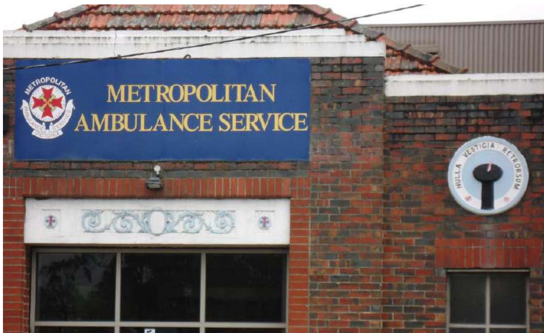
Figure 80. Detail of the station, showing the bas-relief decoration. (Source: Context, 2016)
