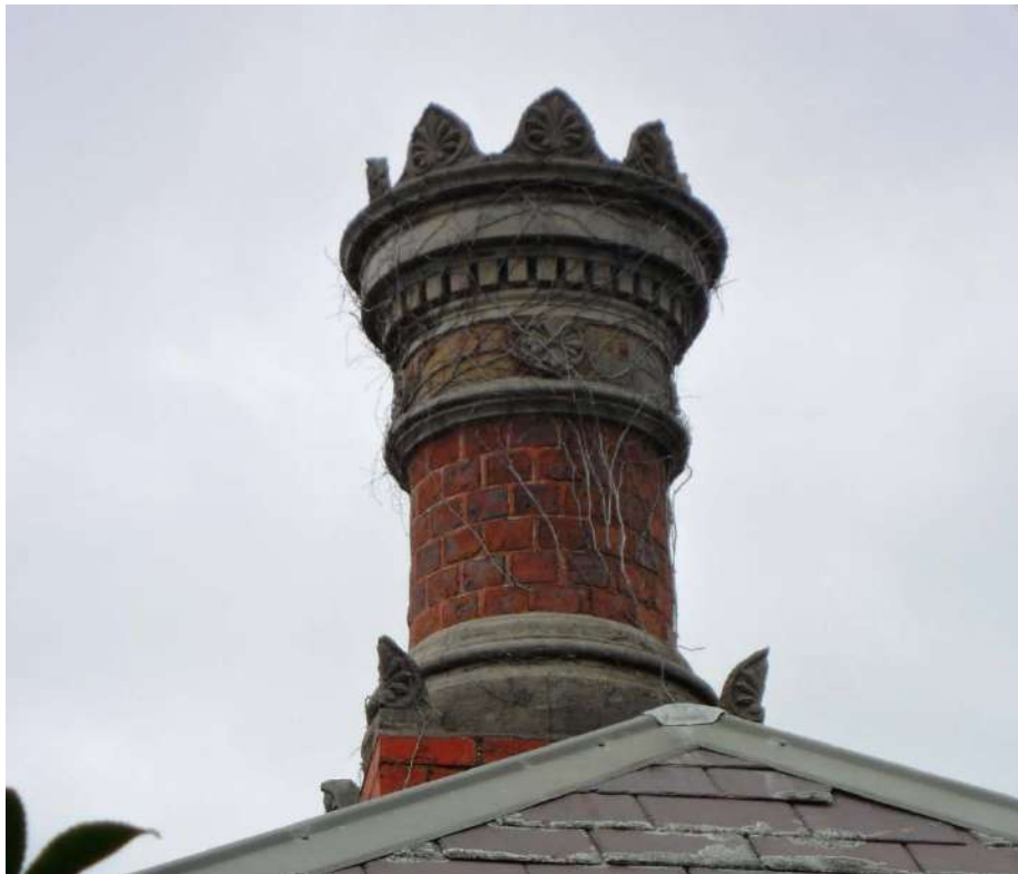
Figure 62. Front chimney. (Source: Context 2016)
