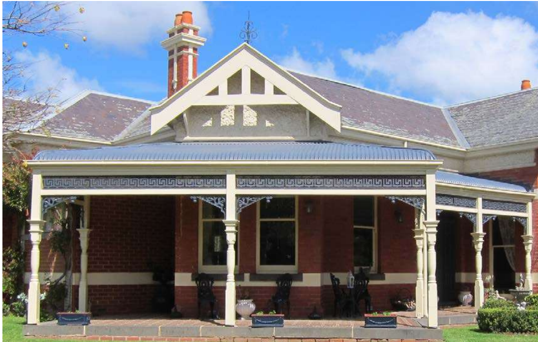
Figure 129. Verandah frieze and chimney at 49 Mangarra Road.
