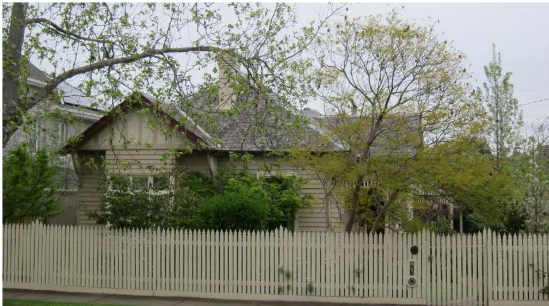
Figure 21. 11 Maling Road. (Source: Context, 2016)
