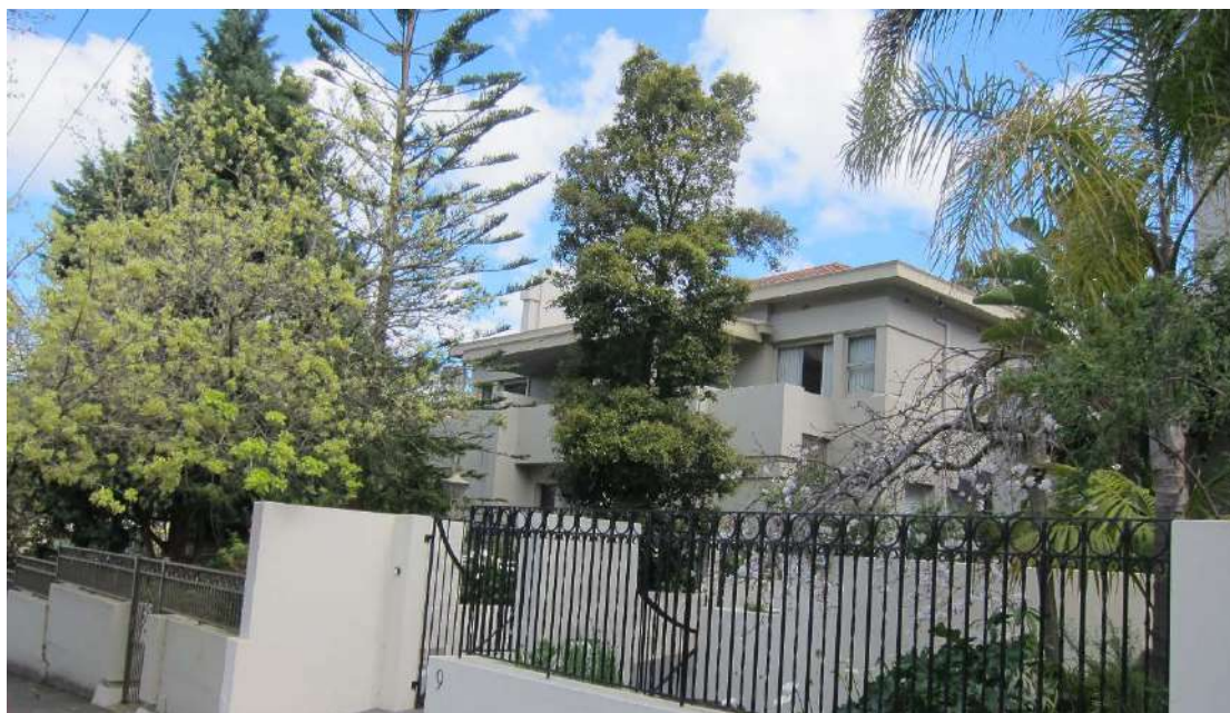
Figure 43. Number 7 Rochester Road (HO184). (Source: Context, 2016)
