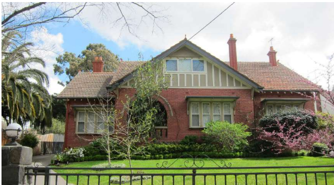
Figure 40. Number 33 Rochester Road. (Source: Context, 2016)
