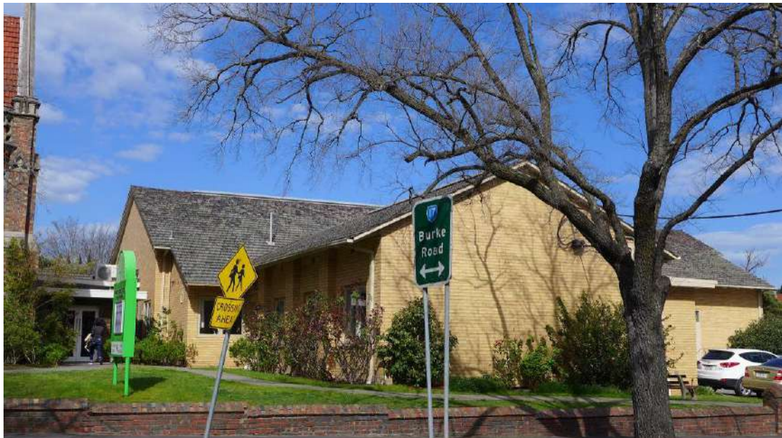
Figure 71. 1958 Church Hall from Mont Albert Road. (Source: Trethowan Architecture 2016)
