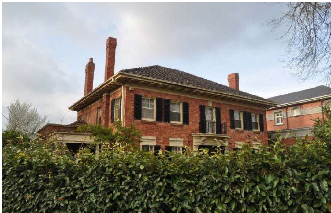
Figure 132. South façade. (Source: Trethowan Architecture 2016)
