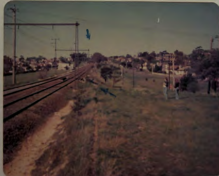
BRIDGE OVER POWER AVE. facing east. Map 2.8 N 7.8 E
